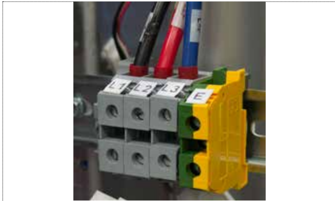
1. Delta Power Supply terminal block.
