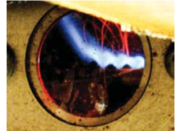
Lifting flame with too much air
